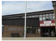
Whitewater Valley Elementary
