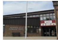
Whitewater Valley Elementary
