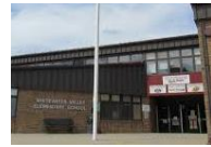
Whitewater Valley Elementary
