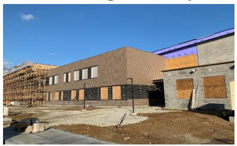
Harrison Junior High: Roof installation continues above the admin area while brick continues along the North wall of Area A. Drywall is being hung on the 2<sup>nd</sup> floor of Area B and finished on the 3<sup>rd</sup> floor of Area A. Painting and ceiling grid installation continues on the 1<sup>st</sup> and 2<sup>nd</sup> floors of Area A. Window installation is complete in the courtyard.
