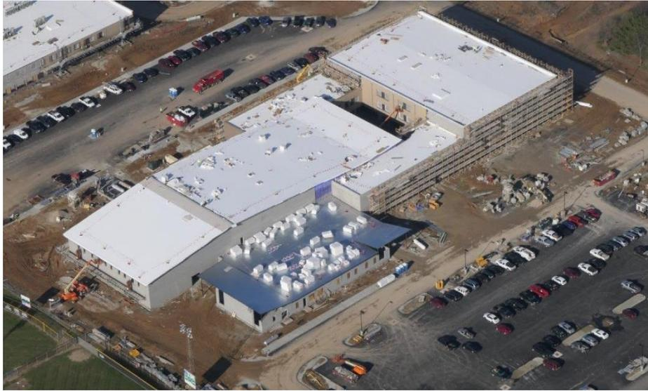
**Harrison Junior High:** Roof installation continues above the gyms and admin area while brick continues along the North wall of Areas A. Drywall is being hung on the 3<sup>rd</sup> floor of Area A and being finished on the 1<sup>st</sup> floor. Painting and ceiling grid installation continues on the 2<sup>nd</sup> floor. Exterior light poles have been installed at the Miami Whitewater / Junior High Campus.
