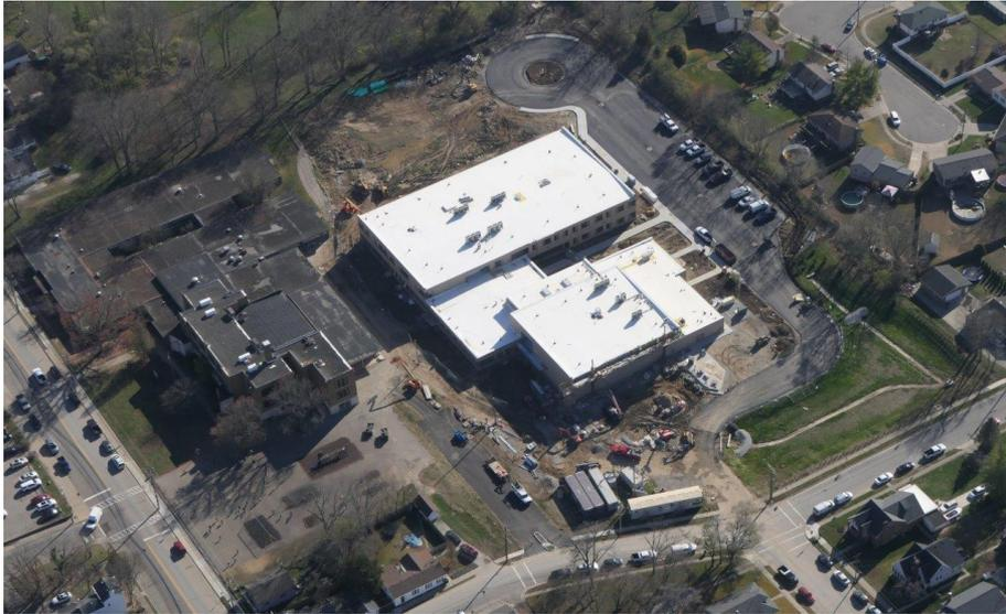
**Harrison Elementary:** In Area A, the administration wing is being painted and ceiling grid installation has begun. Classroom cabinets, windows, and bathroom fixture installation continues throughout Area B. Metal gutters are being installed along the roof while steel has been set for the main entrance canopy. A major project milestone was reached with all 3 sites now having the base coat of asphalt down!
