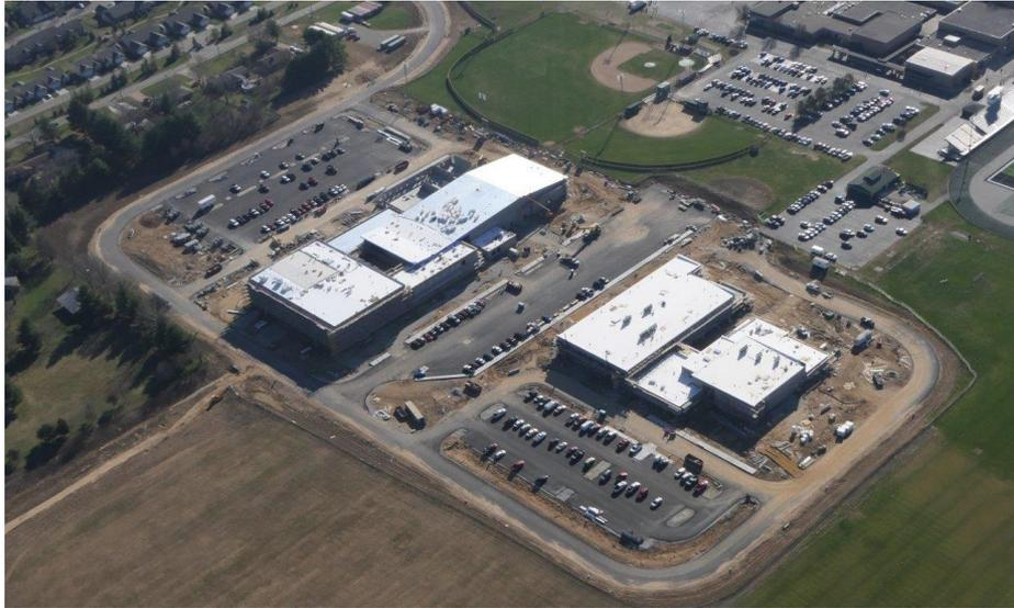
**Harrison Junior High:** Roof steel has been erected above the main gym while roof installation continues over the academic wing. Bearing block walls in the administration wing will be completed this week and brick continues to be laid in the courtyard. The interior walls are framed up on the 3<sup>rd</sup> floor of Area A and 2<sup>nd</sup> floor of Area B. In-wall and above ceiling MEP rough-in continues in all Areas.
