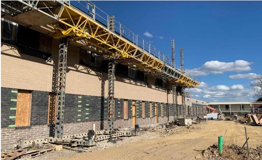
**Crosby Elementary:** The 2<sup>nd</sup> floor of the Area B academic wing has been painted and the ceiling grid is being installed. Classroom cabinet installation has started on the 1<sup>st</sup> floor. The administration area drywall has been hung and drywall finishing has begun. Brick is being laid along the admin roof and the concrete sidewalks are complete along the bus lot. Overhead MEP rough-in continues in both Areas.
