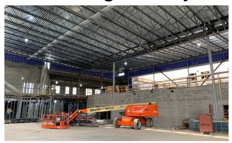
Harrison Junior High: Roof steel erection is complete on the East half of Area A and ongoing above the auxiliary gym while roof installation continues on Areas A & B. Bearing block walls continue to rise in Area C at the main gym and in the administration wing. The interior drywall walls are being laid out on the 3<sup>rd</sup> floor of Area A. In-wall and above ceiling MEP rough-in continues in all Areas.
