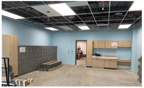
Harrison Elementary: Drywall is being finished in the administration wing while the classroom and gym walls are being painted. Bathroom fixtures and classroom cabinets are being installed on the 1<sup>st</sup> floor of the Area B academic wing. Window installation continues in Area B and metal gutters are being installed along the roof. The kitchen cooler in Area A is being installed. Brick is being laid along the North wall.
