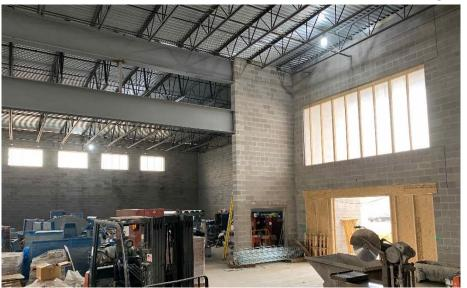
Miami Whitewater Elementary: The interior block walls are nearly complete in Area A and drywall is being hung in the administration wing. In Area B, ceiling grid installation continues on the 1<sup>st</sup> floor while the 2<sup>nd</sup> floor is being primed and painted. MEP rough-in continues in both Areas.
