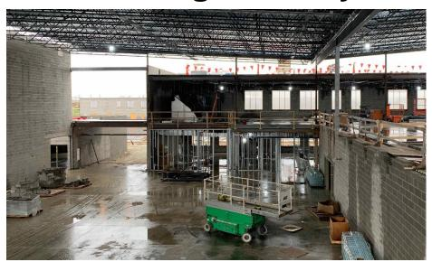
Harrison Junior High: Roof steel is complete on the East half of Areas A & B while roof installation continues on the West half of Area B. Bearing block walls continue to rise in Area C at the main gym and in the administration area. In-wall and above ceiling MEP rough-in continues in all Areas.
