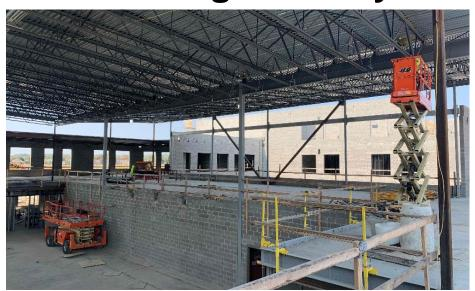
Harrison Junior High: Bearing block walls continue to rise in all 3 Areas while roof steel has been set on the West half of Area B. The bus lot sidewalks are being poured and asphalt paving has begun around the exterior loop road and parking lots. In-wall and above ceiling MEP rough-in continues in all Areas.
