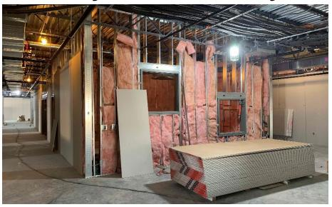
Crosby Elementary: In Area B, drywall is being hung on the 2<sup>nd</sup> floor and finished on the 1<sup>st</sup> floor. In Area A, metal roof decking is being installed above the art room and administration area while interior block walls are being built in the kitchen. Brick is complete outside of the kitchen and mechanical room. In-wall and above ceiling MEP rough-in continues in both Areas.
