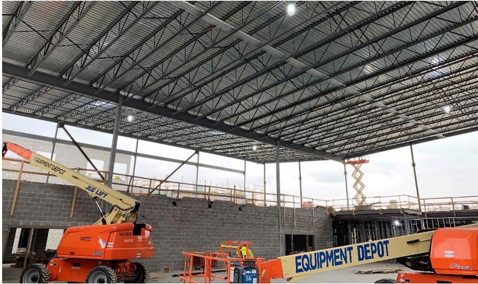
**Harrison Junior High:** Bearing block walls continue to rise in Areas A and C while roof steel is being set on the 2<sup>nd</sup> floor of Area B. The bus lot sidewalks are being poured and stone is being placed at the access roads in preparation for asphalt. In-wall and above ceiling MEP rough-in continues in all Areas.
