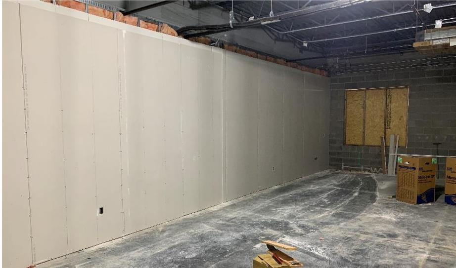
**Miami Whitewater Elementary:** The roof is being installed above the kitchen, mechanical room, administration, and art room in Area A. The interior walls are being laid out and framed in Area A and drywall is being hung on the 1<sup>st</sup> floor of Area B. Brick continues on the East wall of Area B. Above ceiling and in-wall MEP rough-in continues in both Areas.
