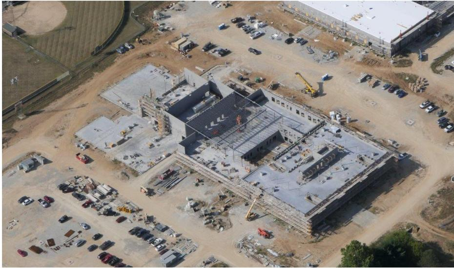
**Harrison Junior High:** Bearing block walls continue to rise in Areas A and C while roof steel is being set on the 2<sup>nd</sup> floor of Area B. Concrete work has shifted from the courtyard to the bus lot sidewalks. In-wall and above ceiling MEP rough-in continues in all Areas and the last DOAS unit has been set in the building.
