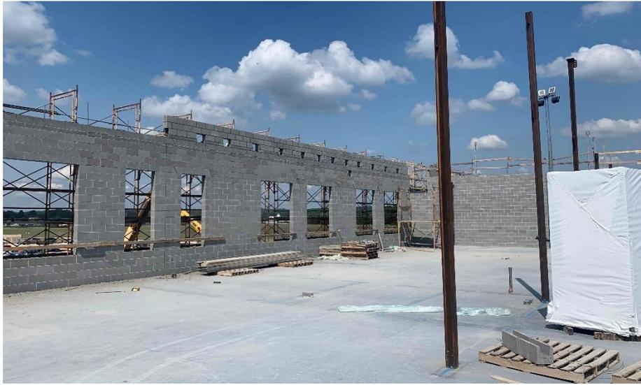
**Harrison Junior High:** In the academic wing, the concrete slab for the 3<sup>rd</sup> floor has been poured which completes all building concrete work for the four Southwest schools! The interior walls on level 2 are being laid out and framed. Bearing block walls continue to rise in Areas B & C while roof steel is being set on the 2<sup>nd</sup> floor of Area B. In-wall and above ceiling MEP rough-in continues in both Areas.
