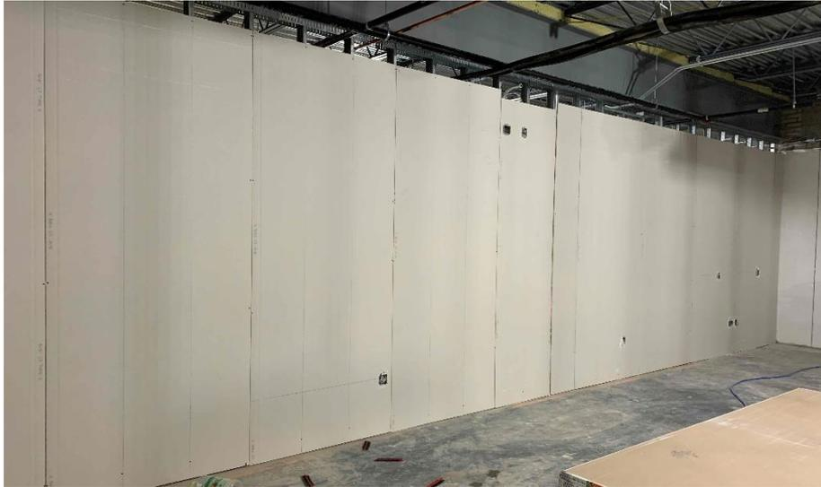
**Crosby Elementary:** In Area B, drywall is being hung in the 1<sup>st</sup> floor and block filler is being painted on the CMU walls. On the 2<sup>nd</sup> floor, interior CMU block walls are being laid around the restrooms and the sprinkler line installation has begun. In-wall and above ceiling MEP rough-in continues in both Areas.
