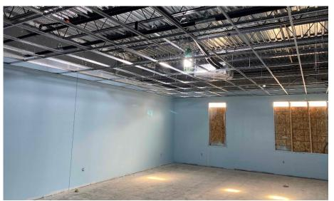
Harrison Elementary: In Area A, structural steel is being erected in the art room and administration area while the roof over the kitchen and mechanical room has been installed. In the academic wing, the 1<sup>st</sup> floor walls are being painted followed by ceiling grid installation while drywall is being hung and finished on the 2<sup>nd</sup> floor. Brick is being laid in the courtyard between Areas A and B.
