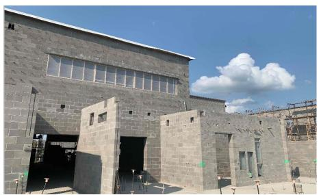
Miami Whitewater Elementary: Bearing block walls are being laid in the kitchen, mechanical room, and administration area in Area A. In Area B, structural steel for the roof is being set in the North half of the 2<sup>nd</sup> floor while the roof is being installed in the South half. The interior walls on the 2<sup>nd</sup> floor are being laid out. In-wall and above ceiling MEP rough-in continues throughout Area B.
