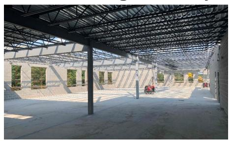
Harrison Junior High: In the academic wing, structural steel is being erected in the East half of the 2<sup>nd</sup> floor. The concrete slab for the 3<sup>rd</sup> floor is scheduled to be poured next week which will complete all building concrete work for the 4 schools. The Area B interior walls are being laid out and framed on the 1<sup>st</sup> floor and the Area C bearing block walls continue to rise in the kitchen.
