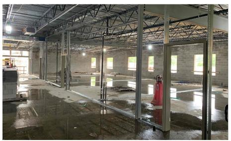
Crosby Elementary: In Area A, the art room bearing block walls will be completed this week while the kitchen is being prepped for structural steel. Roofing installation and the 2<sup>nd</sup> floor interior wall framing began this week in the academic wing. In-wall and above ceiling MEP roughin continues in both Areas.
