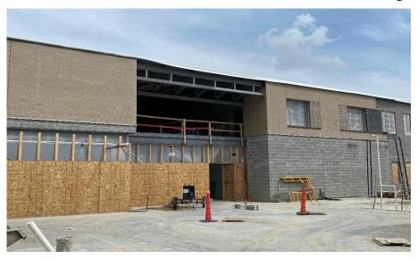
Harrison Elementary: In Area A, brick has been laid at the kitchen and mechanical room wall while bearing block walls are rising in the art room and administration area. In the academic wing, the 1<sup>st</sup> floor walls are being painted while drywall is being hung and finished on the 2<sup>nd</sup> floor. Above ceiling MEP rough-in continues in both Areas.
