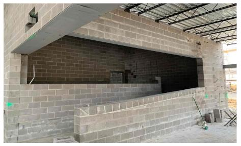
Miami Whitewater Elementary: Bearing block is being laid at the kitchen and administration area in Area A and structural steel is being set at the mezzanine. In Area B, the block walls are being laid up to the roof level in the North half of the 2<sup>nd</sup> floor while roof steel is being set in the South half of the 2<sup>nd</sup> floor. In-wall and above ceiling MEP rough-in continues throughout Area B.
