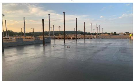
Harrison Junior High: In the academic wing, the 2<sup>nd</sup> floor bearing walls are rising in the East half while structural steel is being set in the West half. The elevated slab in the West half of Area B has been poured and the interior walls are being laid out on the 1<sup>st</sup> floor. In-wall and above ceiling MEP rough-in continues.
