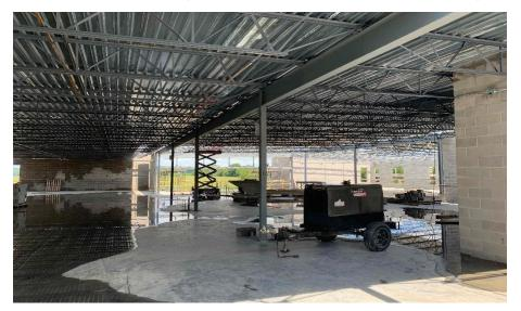
Crosby Elementary: In Area A, bearing block walls are being laid up in the administration area while brick is being laid over the kitchen and mechanical room. In Area B, roof steel and decking is being set above the academic wing. Inwall and above ceiling MEP rough-in continues in both Areas.
