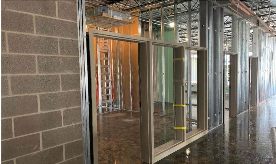
**Crosby Elementary:** In Area A, the metal roof decking is being installed in the gym, cafeteria, and stage. In Area B, the 2<sup>nd</sup> floor block walls are rising to the roof level and the 1<sup>st</sup> floor interior walls and door frames have been framed and set. In-wall and above ceiling MEP rough-in continues in both Areas.
