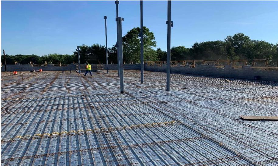
**Harrison Junior High:** The 2<sup>nd</sup> floor of the academic wing has been prepped for next week's elevated concrete pours. Bearing block walls continue to rise in the kitchen and gym in Areas B & C. Metal stairs are being installed in Area A and structural steel is being set in the East half of Area B. In-wall and above ceiling MEP rough-in continues.
