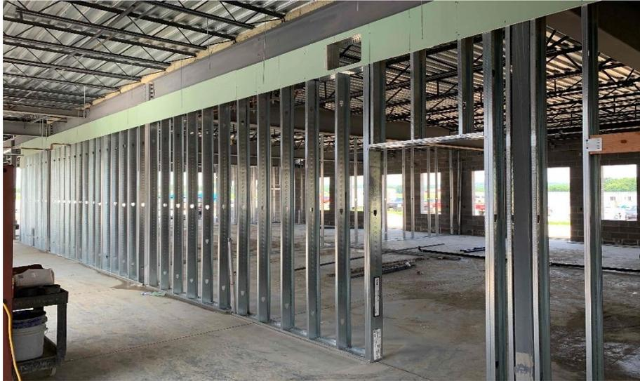
**Miami Whitewater Elementary:** The gym and stage bearing walls continue to rise and the roof steel has been set at the gym in Area A. In Area B, the 1<sup>st</sup> floor interior walls have been framed in and the door frames are being set. The elevated concrete slab in the North half of the 2<sup>nd</sup> floor and the air handling unit concrete pads have been poured. In-wall and above ceiling MEP rough-in continues.
