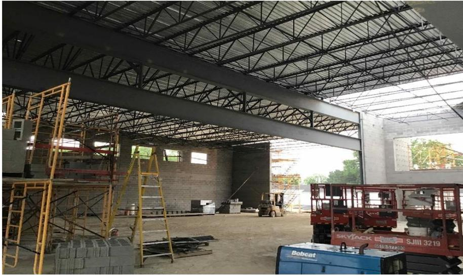
**Harrison Elementary:** In Area A, the gym and mezzanine bearing walls are complete and the mezzanine steel is being set. In Area B, the 2nd floor bearing walls are rising to the roof level, the 2nd floor concrete slabs have been poured, and framing for the 1st floor interior walls has commenced. In-wall and above ceiling MEP rough-in continues in both Areas.
