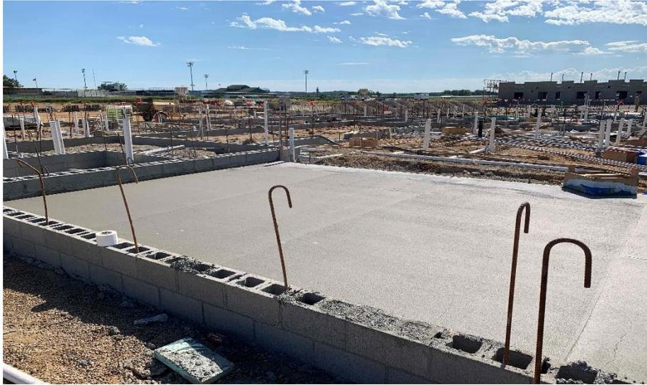
**Harrison Junior High:** In Area A, bearing walls continue to rise along with MEP rough-in for the academic wing, and structural steel sequence #1 has begun. In Area B, the East half of the concrete slab on grade was poured this week and slab prep has begun in Area C. Foundation block also continues in Area C.
