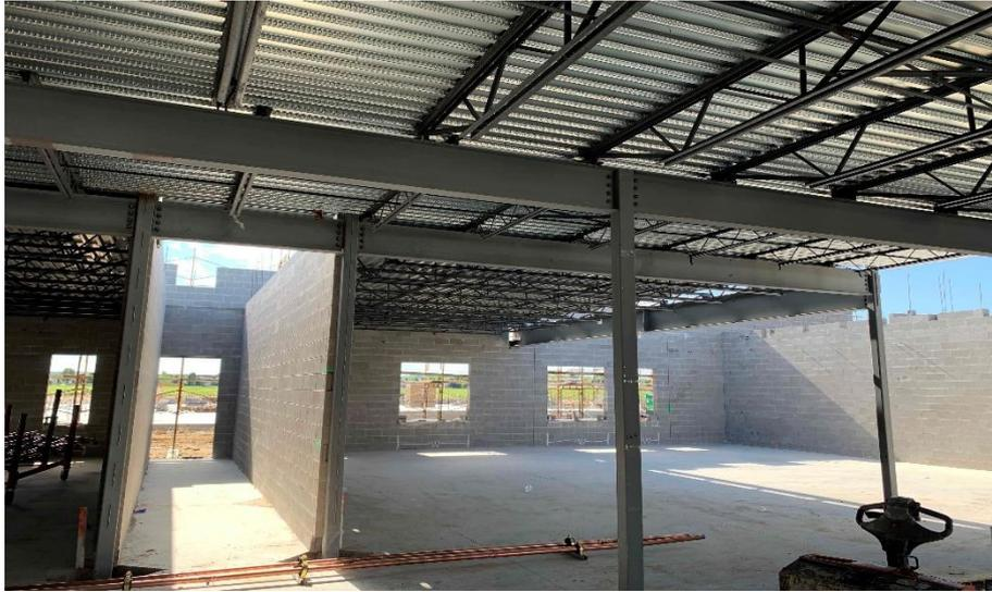
**Miami Whitewater Elementary:** In Area B, the North half of the bearing walls are complete and the 2nd floor steel is being set. Metal decking has been laid on the South half of the 2nd floor and prep for the upcoming elevated concrete slab pour continues. In-wall and above ceiling MEP rough-in continues in both Areas.
