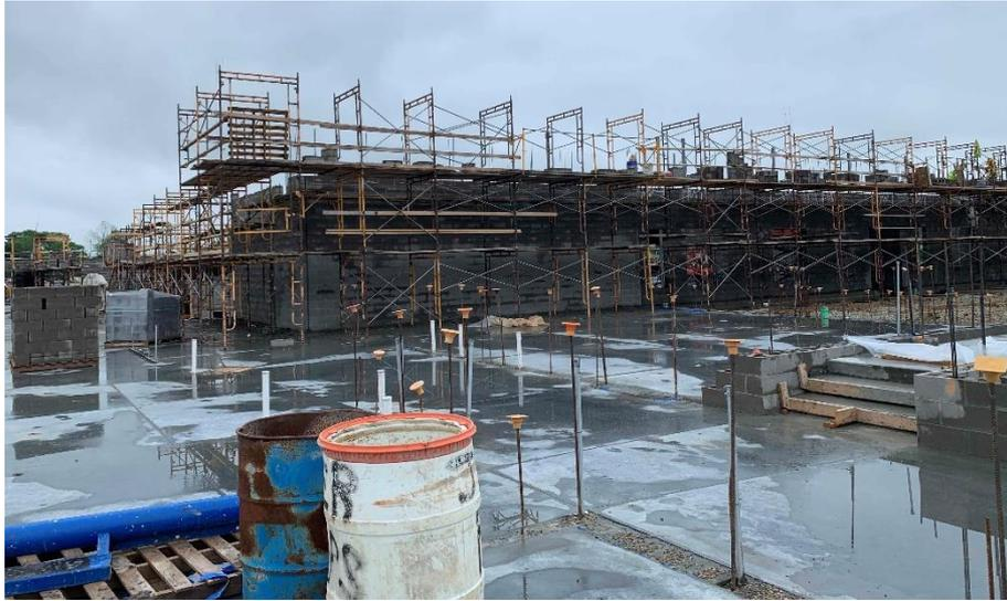
**Miami Whitewater Campus:** 1<sup>st</sup> floor bearing walls in Area B are nearing completion in preparation for 2<sup>nd</sup> floor steel. Steel columns and beams in the South half of Area B have been set and metal decking is being installed. Electrical and plumbing rough-ins are being installed in bearing block.
