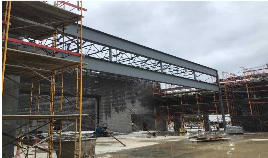
**Harrison Elementary:** The gym, mechanical, and kitchen bearing walls continue to rise in Area A. In Area B, half of the 2<sup>nd</sup> floor concrete slab will be poured this week. The 1<sup>st</sup> floor interior walls are being laid out to start framing next week. In-wall and above ceiling rough-in for MEP piping and duct continues in both Areas A and Area B.
