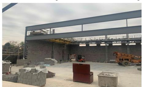
Crosby Elementary: The gym bearing walls are complete and the cafeteria walls continue to rise in Area A. In the South half of Area B, steel is being set for the 2<sup>nd</sup> floor followed by metal decking. Electrical and plumbing rough-ins are being installed in bearing block.
