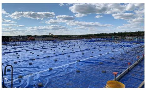
Harrison Junior High: Foundation block continues in Area C while bearing walls are starting to rise in the East half of Area A. The Area B slab on grade is being prepped for next week's concrete pour. MEP underground is being installed in Area C and the parking lot light pole bases are being poured across the site.
