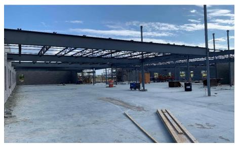
Miami Whitewater Campus: 1st floor bearing walls in the South half of Area B are complete with the North half to follow in preparation for 2nd floor steel. Steel columns and beams in the South half of Area B are being set. Electrical and plumbing rough-ins are being installed in bearing block.
