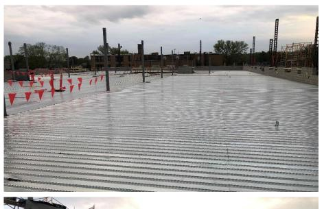
Harrison Elementary: The gym, mechanical, and kitchen bearing walls continue to rise in Area A. In Area B, the 2<sup>nd</sup> floor steel and metal decking will be complete and the concrete slab poured next week. In-wall and above ceiling rough-in for MEP piping and duct has begun in both Areas A and Area B.
