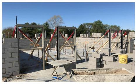
Harrison Junior High: The concrete footers have been completed as foundation block moves from Area B to Area C. Bearing walls have started at the restroom core in Area A while Area B is being prepped for the slab on grade. Underground electric has been installed in Area B and the underground plumbing continues in the kitchen.
