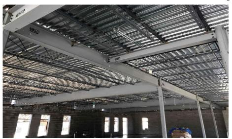
Harrison Elementary: The gym, mechanical, and kitchen bearing walls continue to rise in Area A. In Area B, steel columns and beams are being set in the South half of the 2<sup>nd</sup> floor while the metal decking gets installed in the North half. Electrical and plumbing rough-ins are being installed in bearing block.
