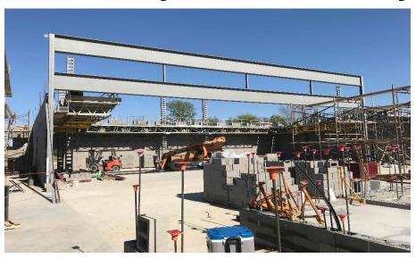
Crosby Elementary: Bearing walls in the gym and the cafeteria continue to rise in Area A. In the North half of Area B, steel column baseplates are being grouted and steel connections are being detailed while metal decking follows closely behind. Electrical and plumbing rough-ins are being installed in bearing block.
