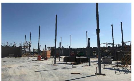
Miami Whitewater Campus: Bearing walls in Area B continue to rise in preparation for the 2<sup>nd</sup> floor steel. The steel columns and beams in the South half of Area B are being set. Electrical and plumbing rough-ins continue in Area B.
