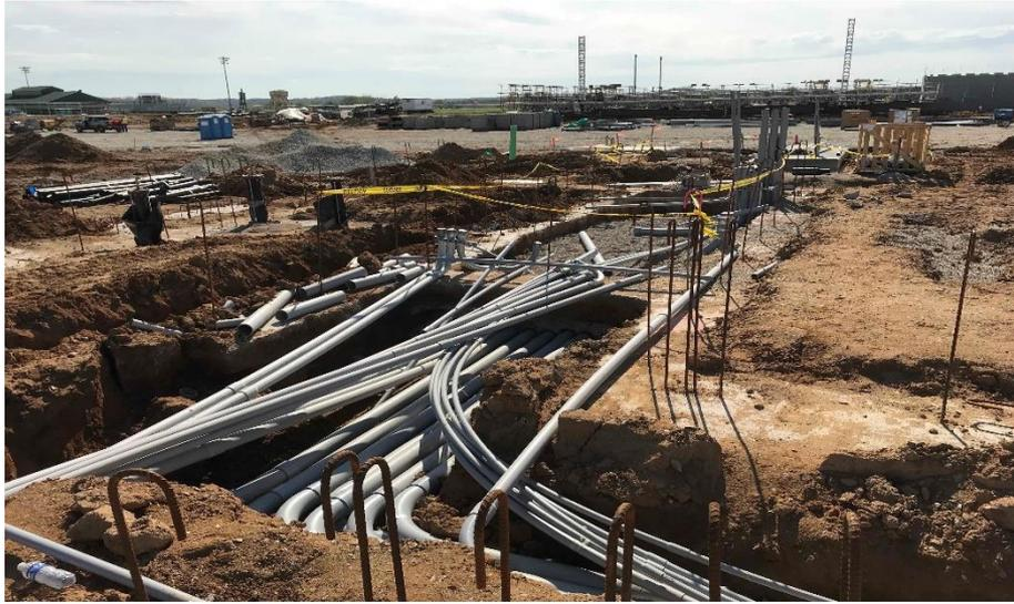
**Harrison Junior High:** The concrete footers in Area C will be complete this week followed by the foundation block in Area B . Underground electric and plumbing is being installed across all 3 areas. In Area A, the East half of the slab on grade was poured last week and the West half will be poured this week.
