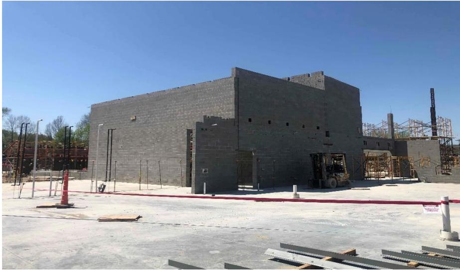
**Harrison Elementary:** The stage bearing walls have been completed and the masons have moved to the gym, kitchen, and mechanical walls in Area A. In Area B, Steel is being set in sequence #2 while the metal decking gets installed in sequence #1. Electrical and plumbing rough-ins are being installed in bearing block.
