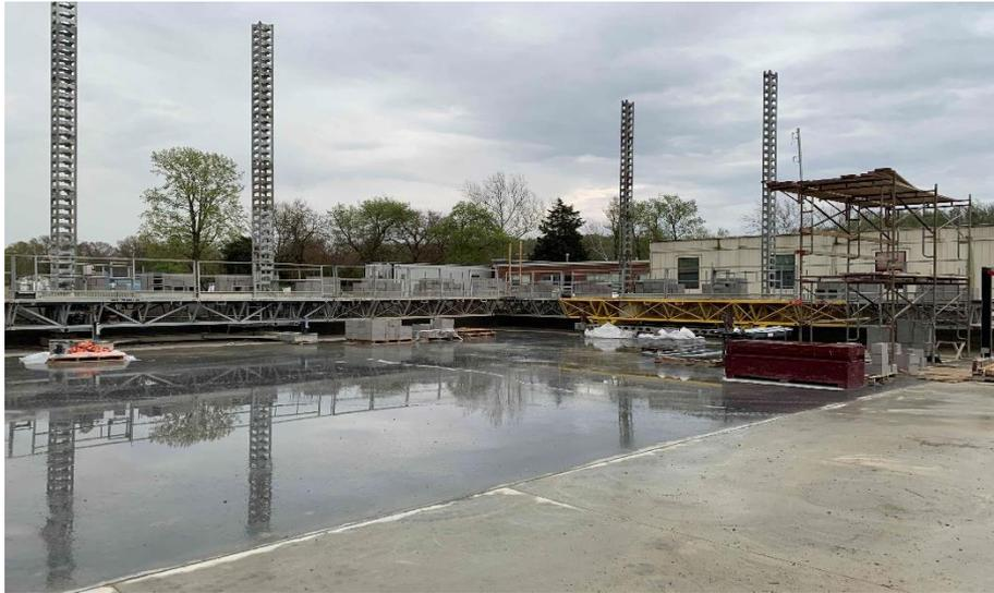
**Crosby Elementary:** Bearing walls in Area A begin to rise with the start of the gym. The stage and cafeteria walls have been laid out this week. In Area B, steel in sequence #1 is being set with metal decking closely behind. Electrical and plumbing rough-ins are being installed in bearing block.
