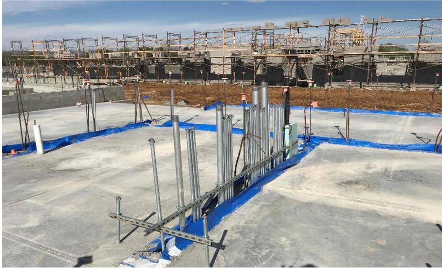
**Miami Whitewater Campus:** Bearing walls in Area B continue to rise in preparation for steel sequences #1 and #2. The site has been prepped for the delivery of steel and the crane. Electrical and plumbing rough-ins continue in Area B. The installation of the gas main across the MWW Elem and the Junior High site continues.
