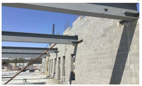
Harrison Elementary: The Area A stage and admin bearing walls continue to rise. The kitchen and mechanical slab on grade has been poured which completes the 1<sup>st</sup> floor building slabs. Steel has been delivered and is being set in Area B to kick off Sequence #1.
