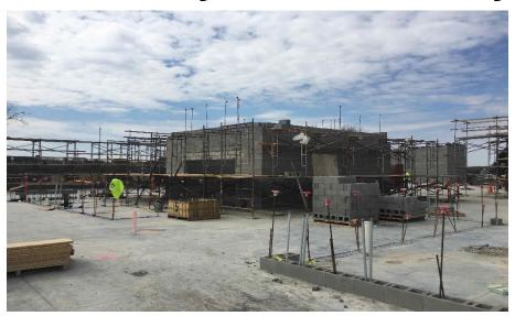
Crosby Elementary: Bearing walls in Area B continue to rise with the completion of the West wall. The Area B elevator and core walls have been laid out. The kitchen and mechanical room slab on grade was poured this week. Electrical rough-ins on exterior walls and plumbing carriers are being installed.
