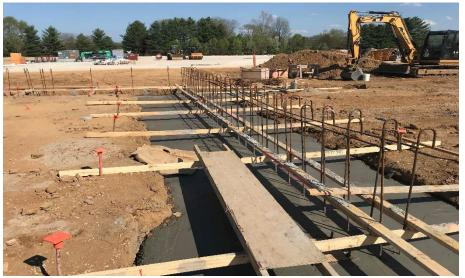
Harrison Junior High: The Area B concrete footers continue South towards Area C. The underground plumbing in Area A will finish this week and move to Area B while the primary electrical conduit is being installed in the electrical room. Foundation block is slated to begin next week in Area A
