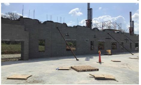
Harrison Elementary: The Area B 1<sup>st</sup> floor North / East bearing wall has been completed and focus has shifted to the Area A stage and admin bearing walls. The kitchen and mechanical slab on grade has been prepped for next week's pour.
