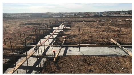
Harrison Junior High: The concrete footers are finishing up in Area A and will move into Area B. The primary electric and site communication feed continue across the site. The main water and fire risers have been installed. The underground MEP is slated to begin in Area A next week.
