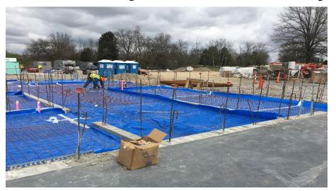
Crosby Elementary: Bearing walls in Area B continue to rise. The gym slab on grade was poured this week and the kitchen / mechanical slab on grade is being prepped for next week's pour. The underground MEP in the kitchen has been completed.
