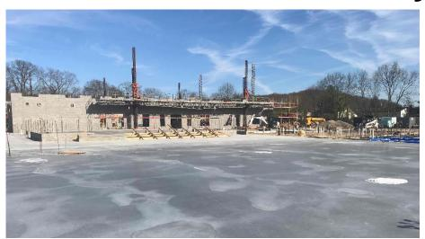
Harrison Elementary: Bearing walls in Area A and Area B continue to rise. The gym slab on grade was poured this week and the kitchen / mechanical slab on grade is being prepped for next week's pour. The underground MEP in the kitchen has been completed.
