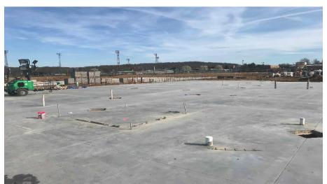
Miami Whitewater Campus: The North half of the Area B slab on grade was prepped and poured this week. In Area A, the underground MEP has been completed while the Foundation CMU continues.
