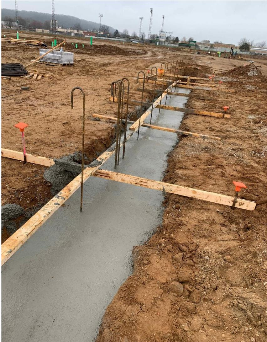
**Miami Whitewater Campus:** The parking lot between the two schools has been stabilized. The concrete footings are finishing up in Area A while the Foundation CMU continues in Area B. Underground MEP will move from Area B to Area A. Our first slab pour is slated for next week!
