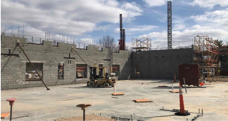
**Harrison Elementary:** Bearing walls in Area B continue to rise. The slab on grade at the Dining and Admin Area has been poured and the prep has begun for the Gym slab. The underground MEP in the kitchen continues. Foundation CMU begins in the kitchen and restroom core.
