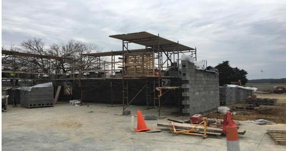
**Crosby Elementary:** Bearing walls in Area B continue to rise. The slab on grade at the Stage and Admin Area has been poured and the prep has begun for the Gym slab. The underground MEP in the kitchen has been completed.
