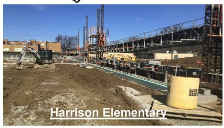
Miami Whitewater Campus: The aggregate piers have been installed at both schools and the concrete strip footings have started at the elementary. Crosby / Harrison El.: Bearing walls continue to rise while the slab on grade prep and underground MEP continue in Area B. The first slab pour is next week!
