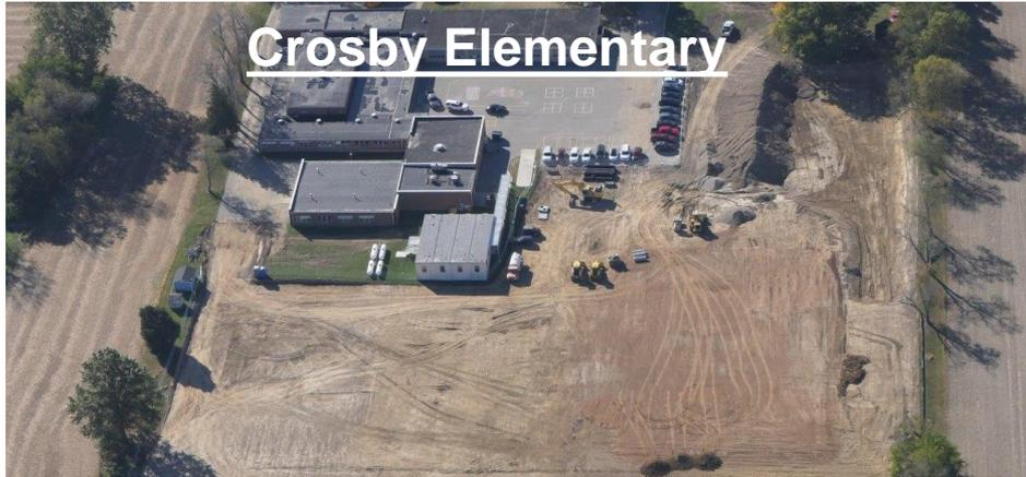
**All Schools:** Mass excavation and grading have been completed at all sites, and the building pads, parking lots, and roads have been cement stabilized. Installation of utility piping for storm water drainage, sanitary waste, and water distribution continues.
